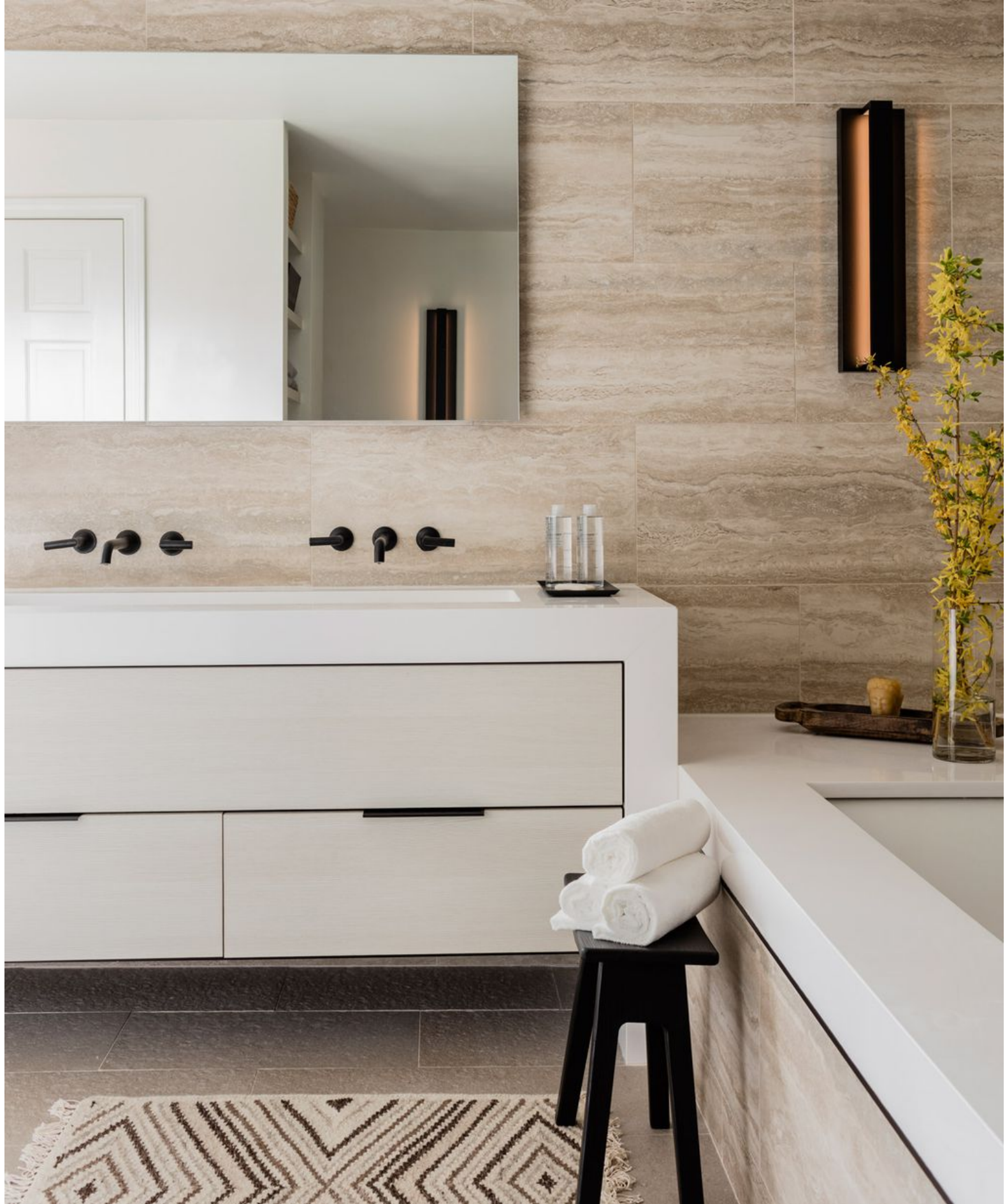
The three-year-long project included redesigning the master bath with clean lines and contemporary finishes. Oversize porcelain wall tiles resemble travertine and the floor has radiant heat, while matte black wall-mounted plumbing fixtures make cleaning the Silestone countertop a snap. MICHAEL J. LEE
